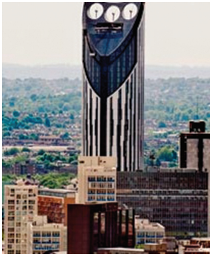
Figure 2. The Strata SE1 Apartment flow analysis: (a) photo from the rear of the wind turbines; and (b) contour plot of wind speed on a horizontal cross-sectional plane (top) and streamlines passing through holes (bottom; CFD by the authors).
